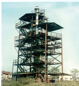
30 tpd v.s.k cement pilot plant at RRL (NEIST)
