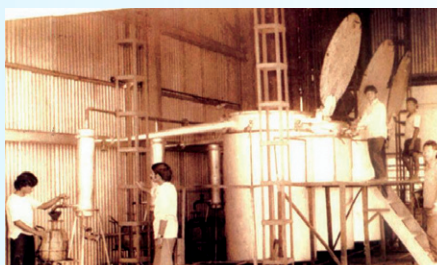
Distillation plant in Yaongyimsen
