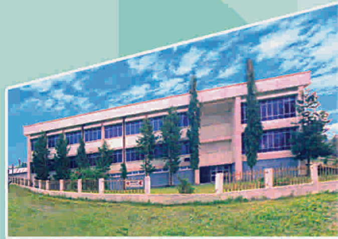
NEIST Branch, Naharlagun, Arunachal Pradesh
