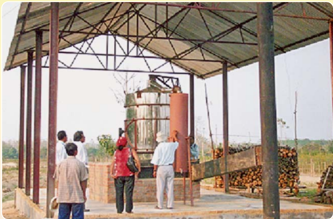
A distillation still under construction and set up by Mrs K Nihokhu Chophi at Nuiland, Dimapur
