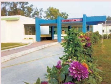
Front view of the facility
