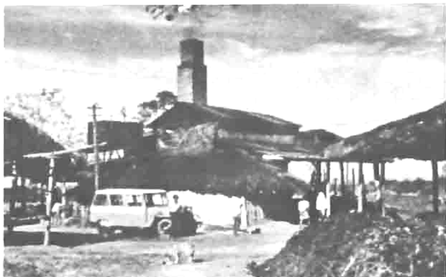
Once there were around sixty distillation plants like this in Pengeri area of Upper Assam
